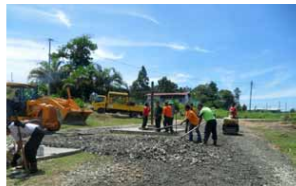
Levelling the parking area by laying stones with compaction machine
